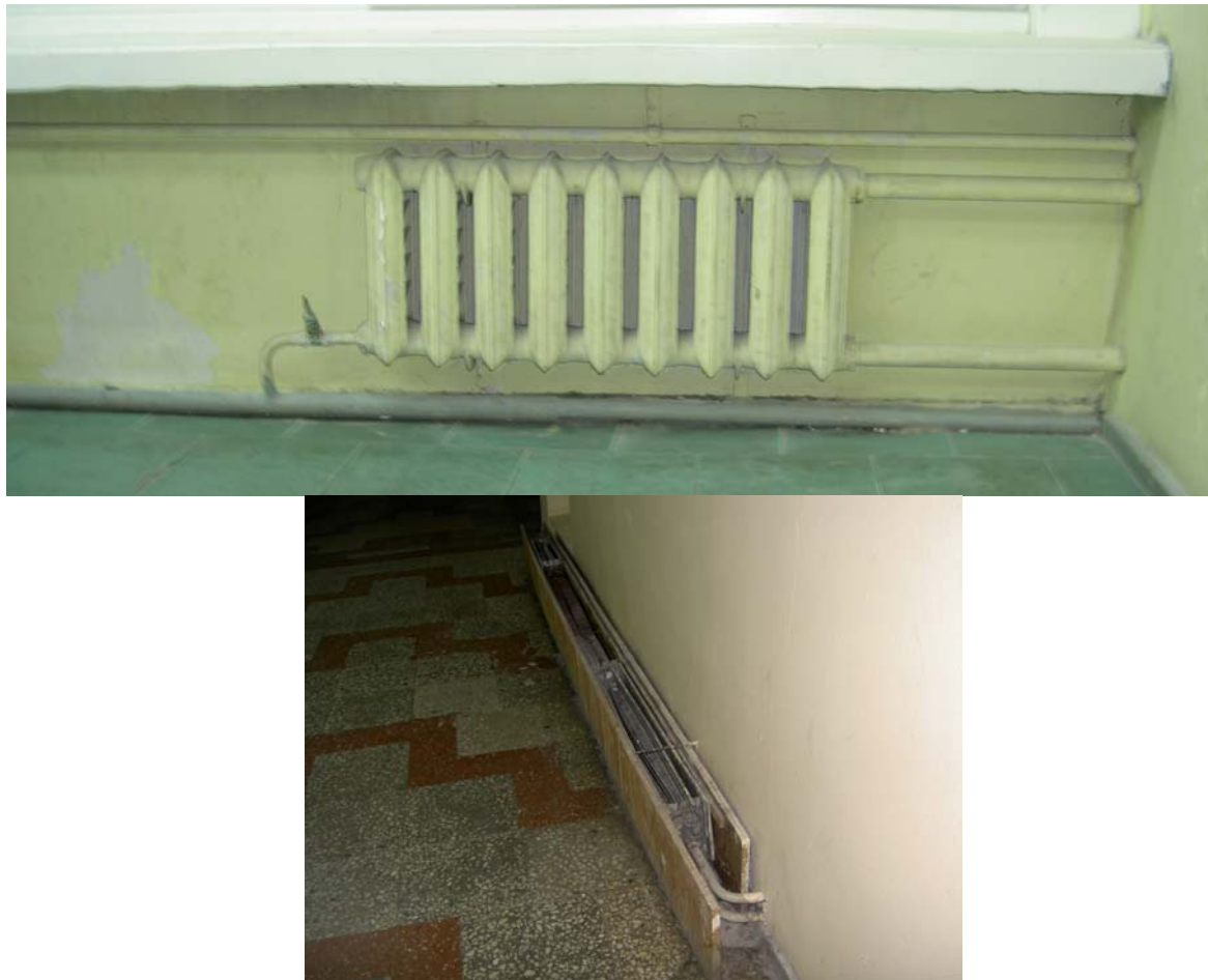
Fig. 5. The sectional radiators M-140 AO and convector heaters in lobbies of the Main building of VGTU
