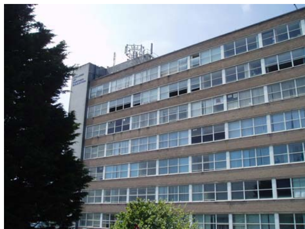
Little or no soffit at roof level to shield building facades
