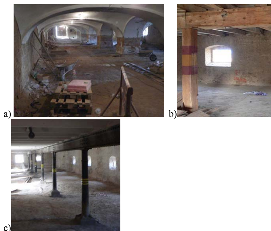
Fig. 7 Ceiling types in the Brewery
