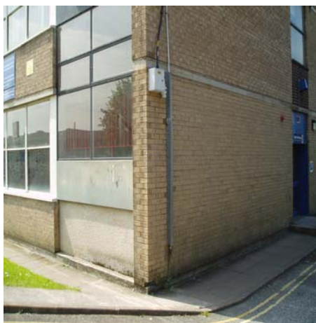
Mortar and brick deterioration at base
