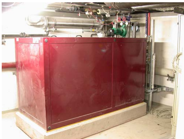
Figure 9 Combined heat and power unit
