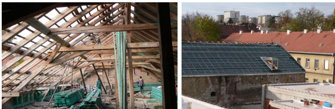
Fig. 9 Conversion of the attic into habitable space
