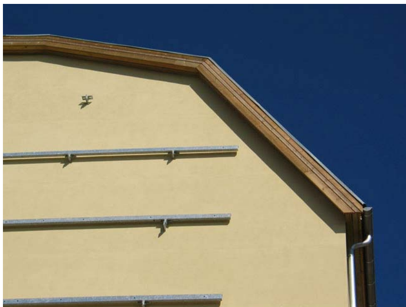
Fig. 10 Mounting racks for the PV-panels on the south gable wall
