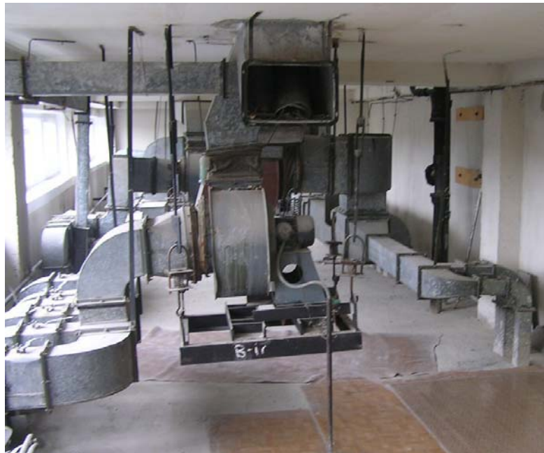
Fig. 8. View of the old mechanical air supply/removal systems in not use in the Main building
